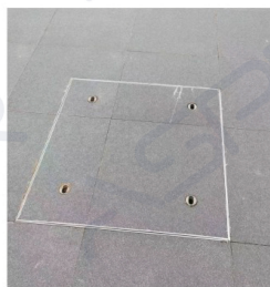
提拉柱井盖安装后
